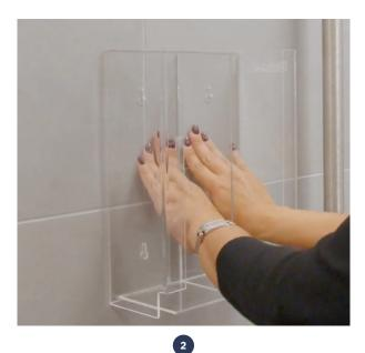
Install bottom of dispenser 42" from floor adjacent to toilet paper dispenser for ADA compliance. Press acrylic holder firmly against wall for over 30 seconds to secure the tape and remove any air bubbles from tape.
